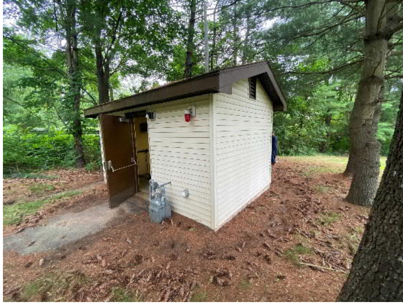
Morgan Street Pump Station: Pump House
