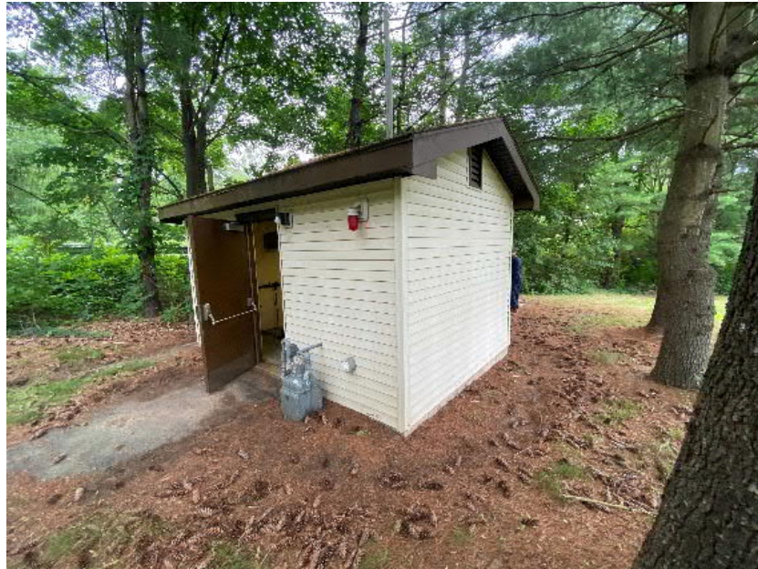
Morgan Street Pump Station: Pump House
