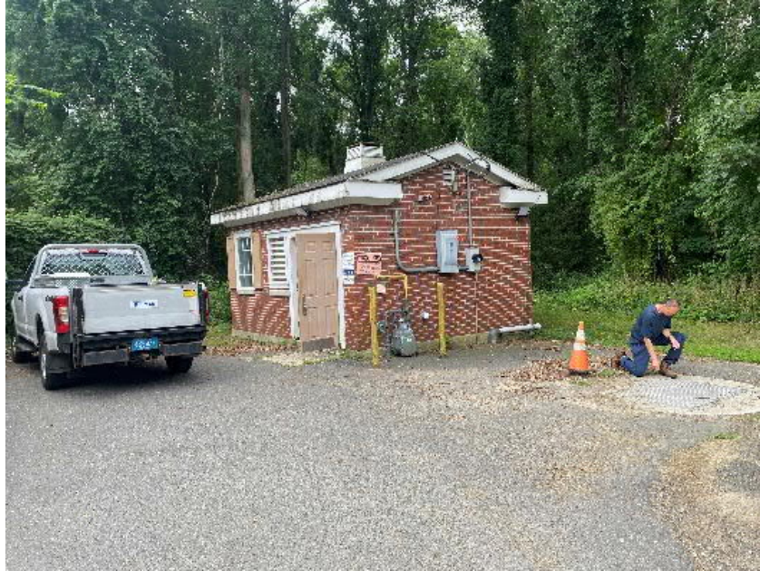
Stony Brook Pump Station: Pump House.
