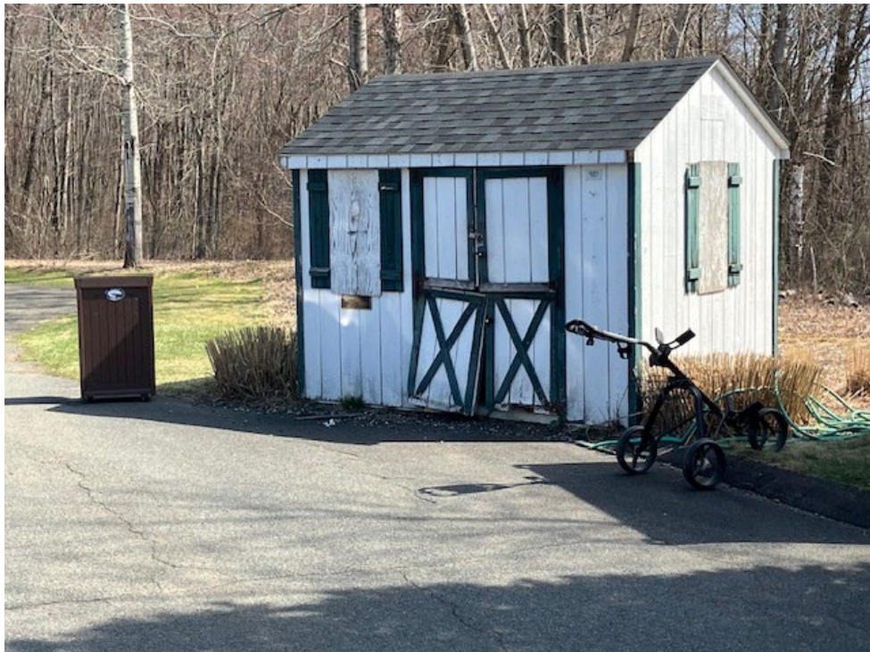
Starter's Hut near #1 tee—prior to recent renovation
