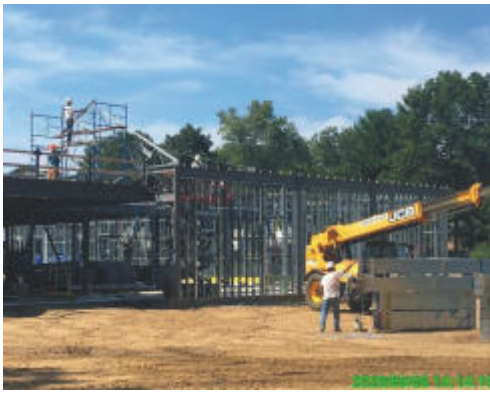
East elevation CFMF complete and installation of roof trusses.
