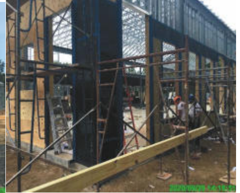
Southeast corner: sheathing and window blocking.
