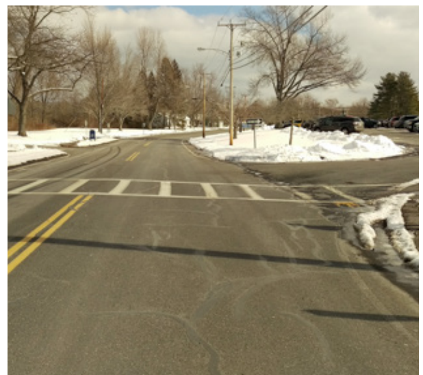
Roadway leading towards school
