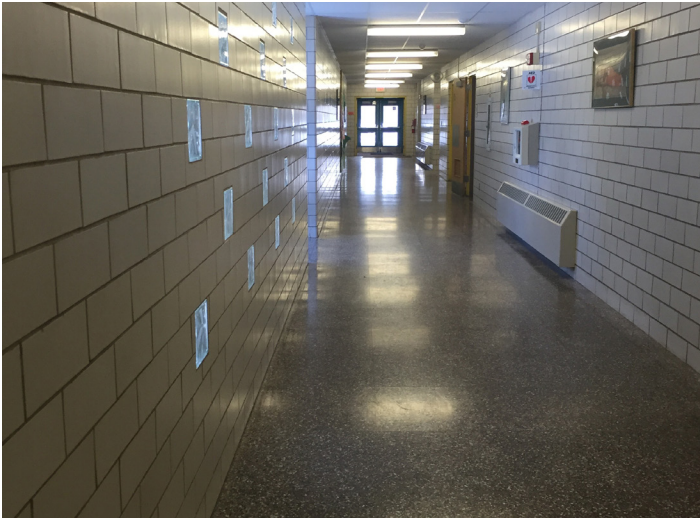
Flooring in corridor
