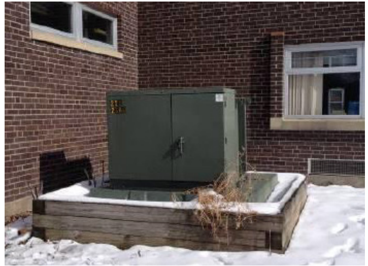
Pad-mounted transformer
