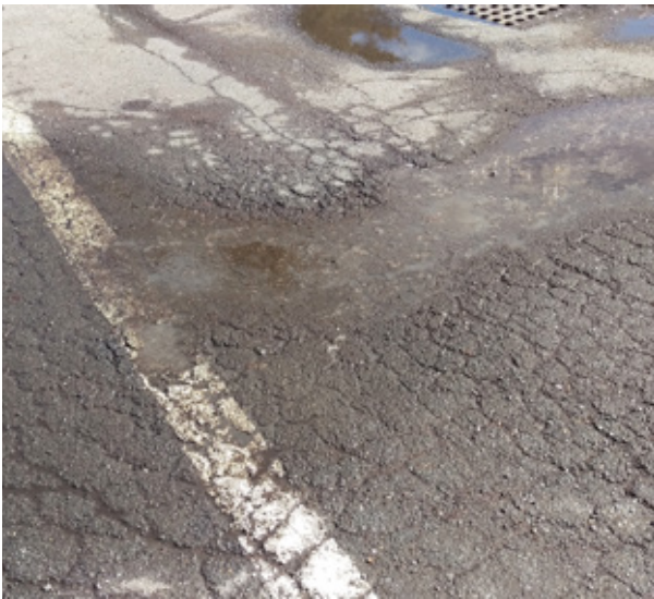
Pavement in parking lot
