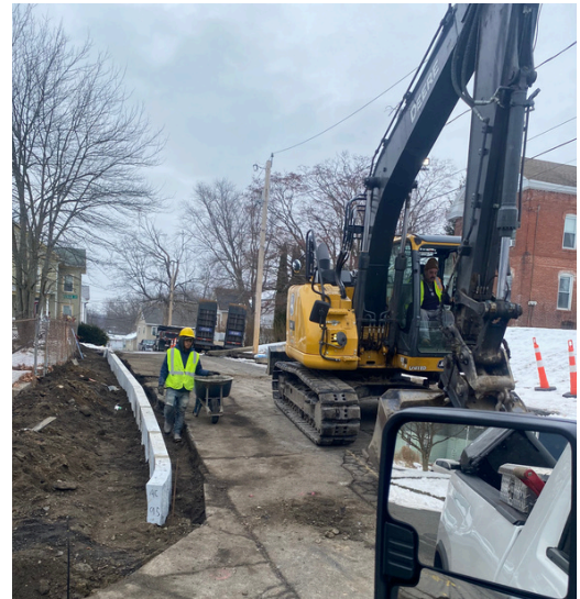
Construction on Graves St.
