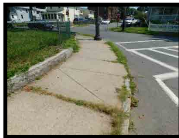
Photo Main Curb Ramps 2
