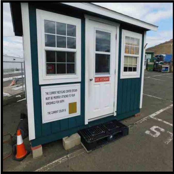
Photo Transfer Station 1
