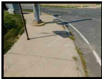
Photo Newton Curb Ramps 5
