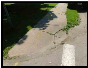
Photo Main Curb Ramps 1
