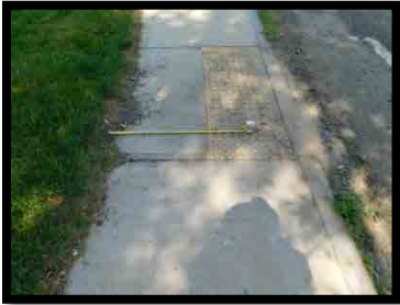
Photo Newton Curb Ramps 4
