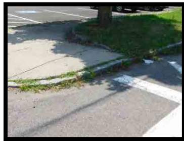
Photo Main Curb Ramps 5
