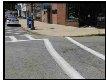
Photo Main Curb Ramps 6
