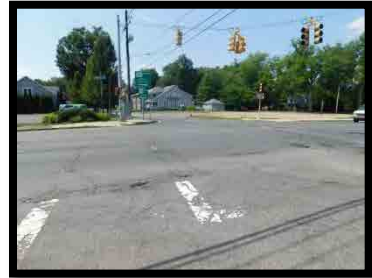
Photo Newton Curb Ramps 6
