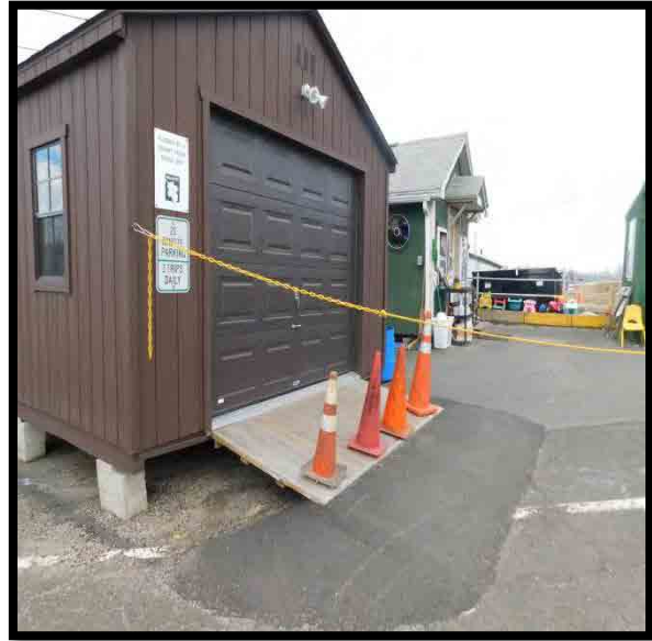
Photo Transfer Station 2
