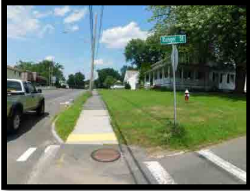
Photo Newton Curb Ramps 1
