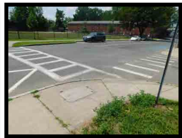
Photo Main Curb Ramps 3
