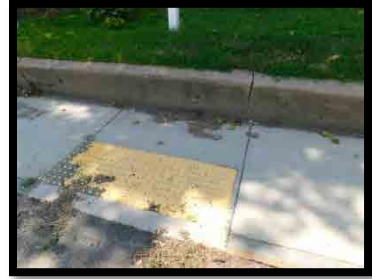
Photo Newton Curb Ramps 3
