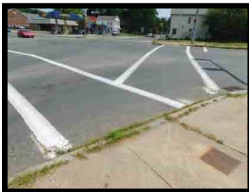
Photo Main Curb Ramps 4
