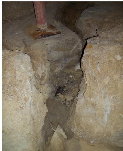
The drain clean-out will be cleaned out (got to love that idea), repaired and the shifting sand and gravel will be returned to its proper resting place. It is easy to see at the base of the lolly-column, how quickly rust is eating away at the flange support of the column due to the high water table. The erosion problem is in the northeast section of the center (away from Dayton and to the left rear when facing the building).
