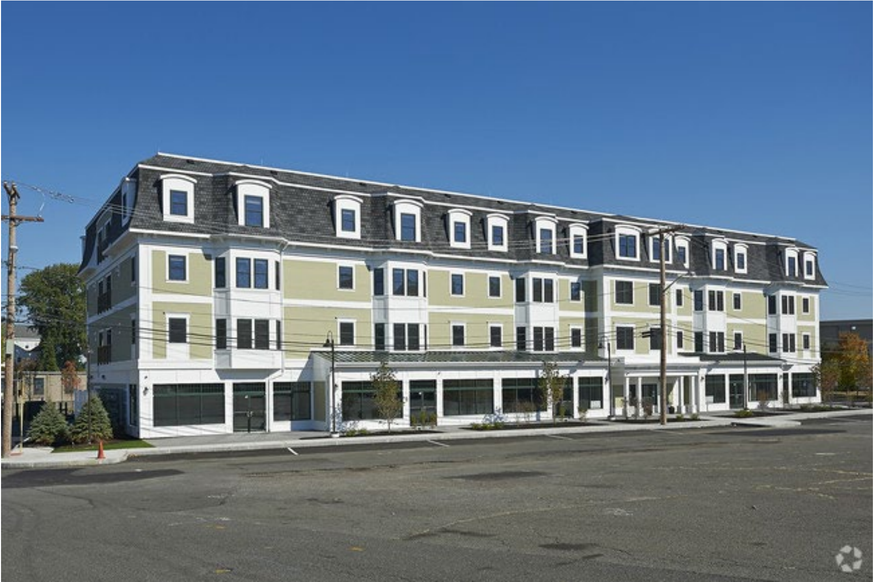
North River Apartments | Salem, MA
