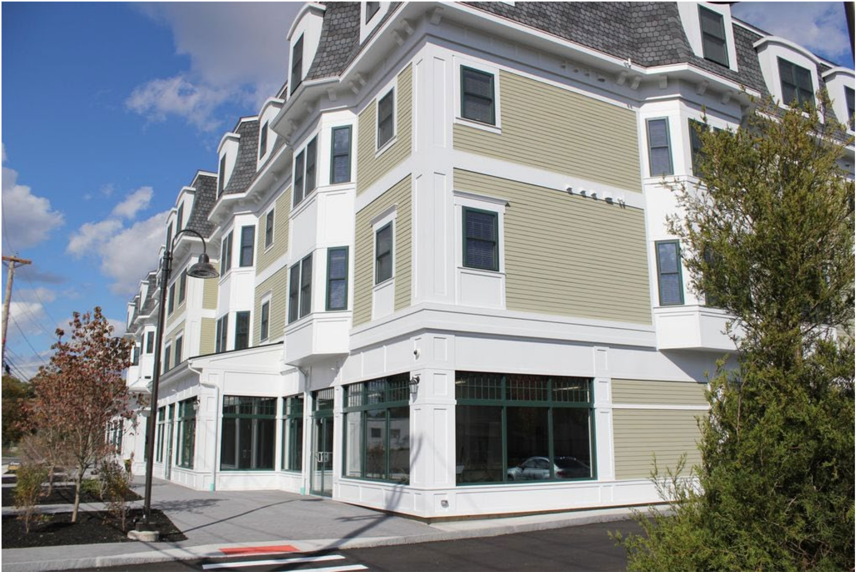
North River Apartments | Salem, MA
