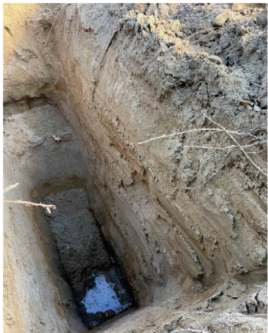
T-1 side wall
