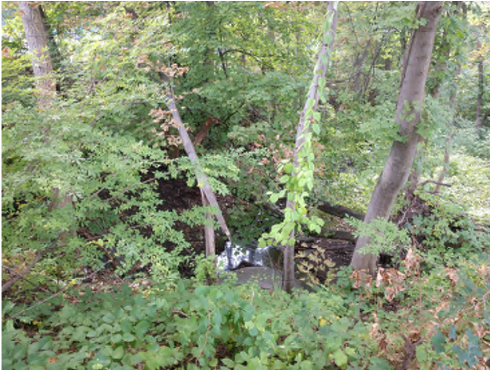
Buttery Brook Culvert outlet
