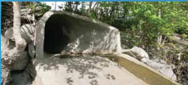
Storm Drain Outfall
