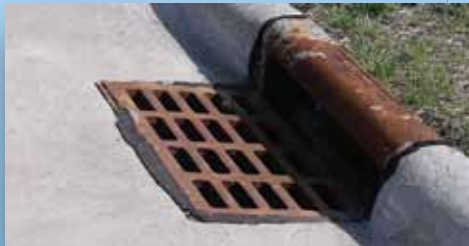
Storm Drain / Catch Basin
