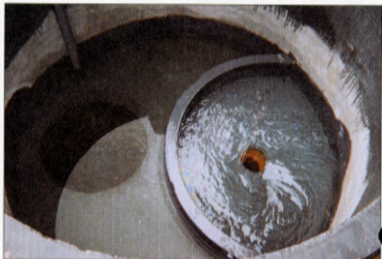
PLATE 3: A view inside the bypass chamber during tests with organic sediment additions, revealing the bypass overflow weir, the small diameter inlet and large diameter outlet pipes from the treatment chamber.
